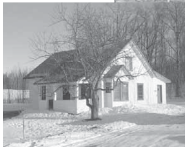
Left: The NOLS Alaska Berry House prior to renovations. Right: Renovations are currently well underway!
