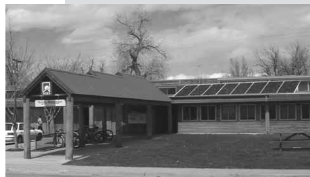
Creative Energies outfitted the NOLS Bus with solar panels three years ago (top) and will now design solar arrays for NOLS Rocky Mountain with a grant from Rocky Mountain Power (bottom, artist's rendition).
